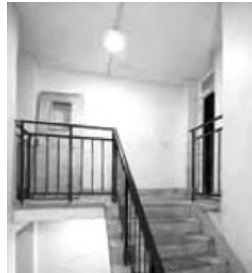
photo of stairwell with LED fitting
