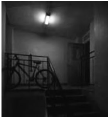
photo of stairwell with fluorescent fitting
